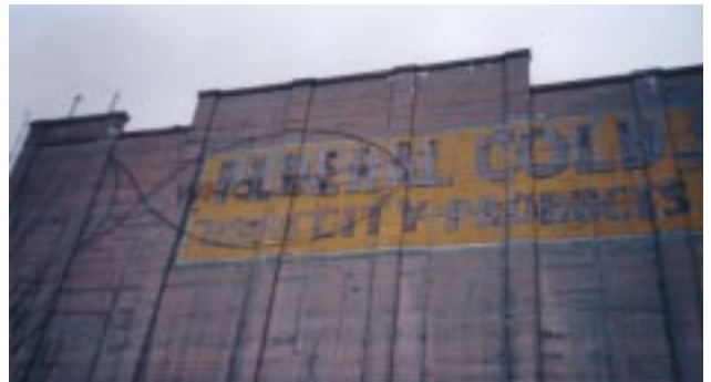
Wholey's Cold Storage Building.
